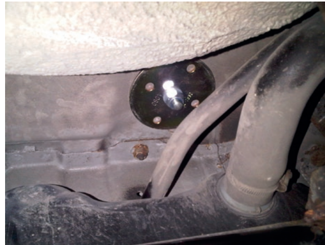
Spreader plates fitted under car floor
